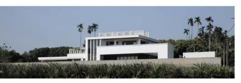
In this design of the building, the length is 30 meters and the center is the main two-story building, the use of overlapping, composition and fusion composed by extending the right level of secondary space 16 meters times 3.5 meters outdoor rain shelter and the left side is 12 m long steel garage ceiling to form a horizontal long white building massing.
